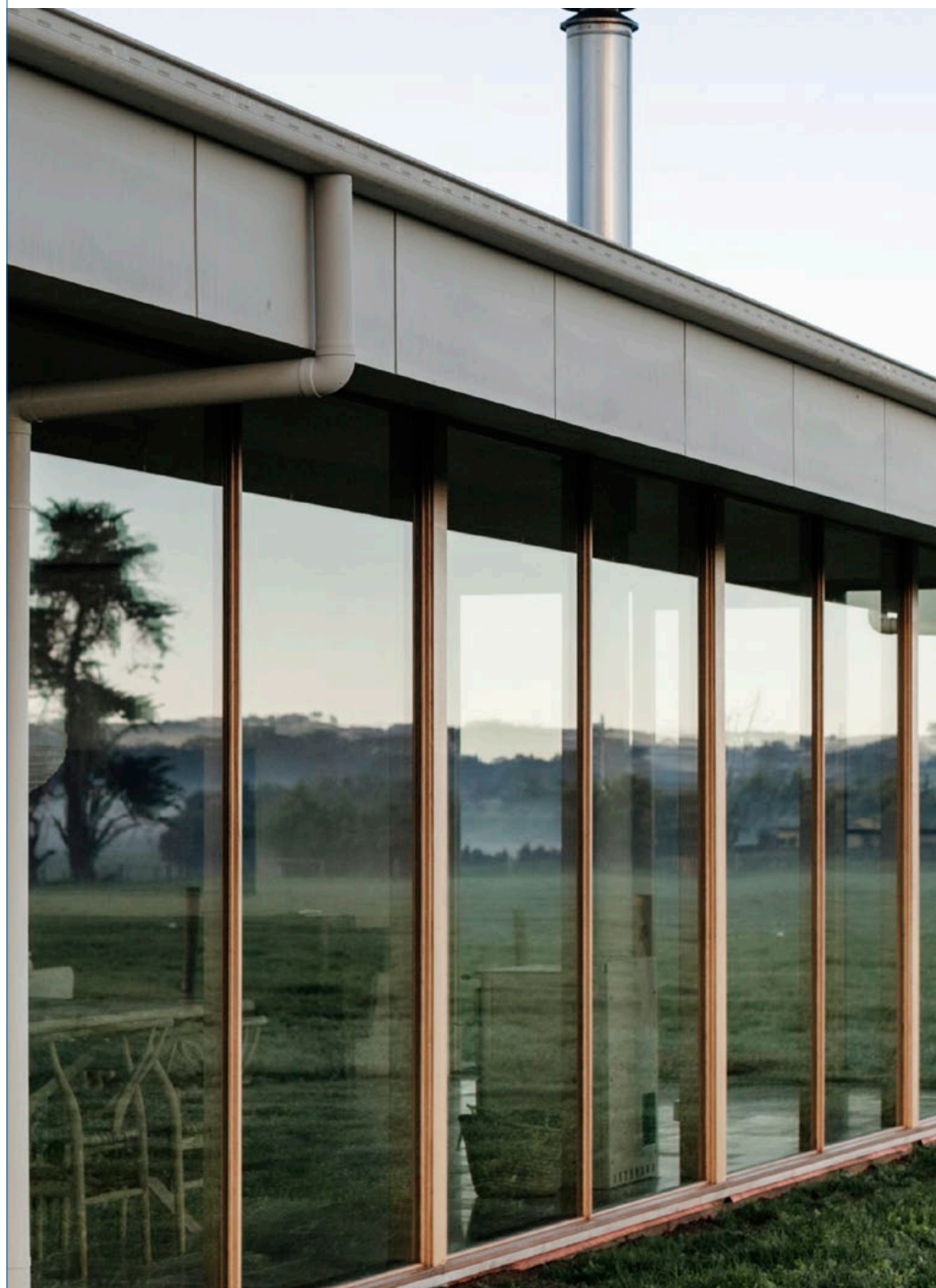
Front cover: Backlit wall, New Zealand | This page: LowE double glazing, Australia
