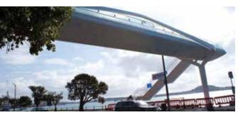
AN EXISTING BRIDGE, BUILT IN THE 1930'S WAS SUFFERING STRUCTURAL FATIGUE. AND WITH THE IMMINENT ELECTRIFICATION OF AUCKLAND'S RAIL NETWORK, THE BRIDGE NEEDED TO BE RAISED.
